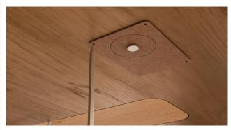
Underneath the surface, use the second magnet with the cardboard template to correctly position the template, use a pencil to mark the screw hole locations.
